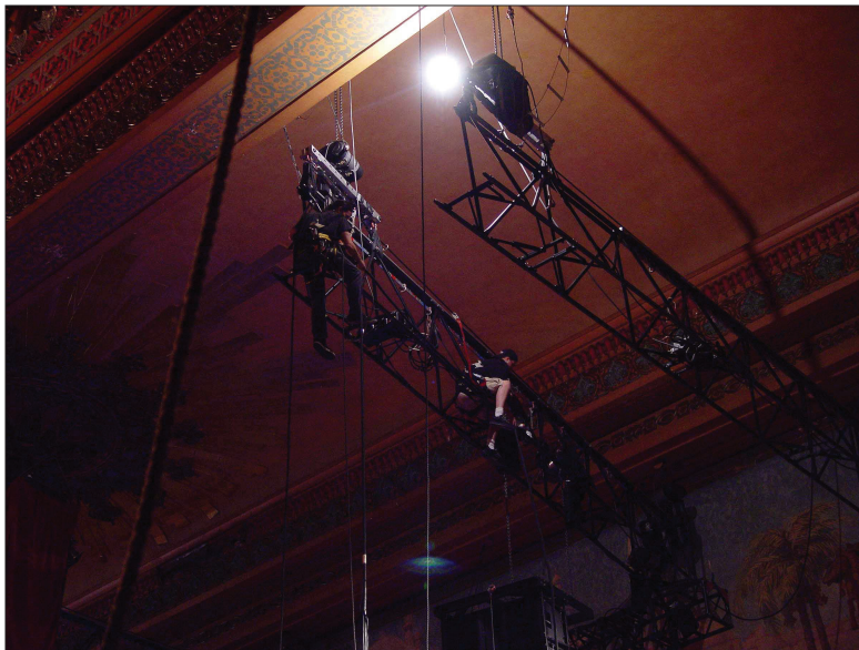
Figure 2.132 Large entertainment shows often require many lights, and possibly the installation of lighting grids. This requires the use of riggers, a term originally coined for people who worked with sailing ships' rigging, but that now includes people who work at heights.
