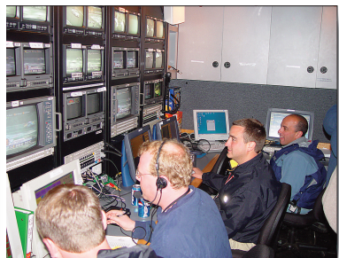
Figure 2.147 Another truck interior, and another vendor of sophisticated graphics. This Sportvision truck with crew of six collects telemetry from race cars and various camera's pan/tilt/zoom positions, mixes in the cars' GPS positions, and produces keyed tags that are automatically placed on the screen near a car as it is viewed by any of the telemetry equipped cameras. These tags contain various information about the cars, and allow viewers to easily identify their favorite car if it is being televised.
